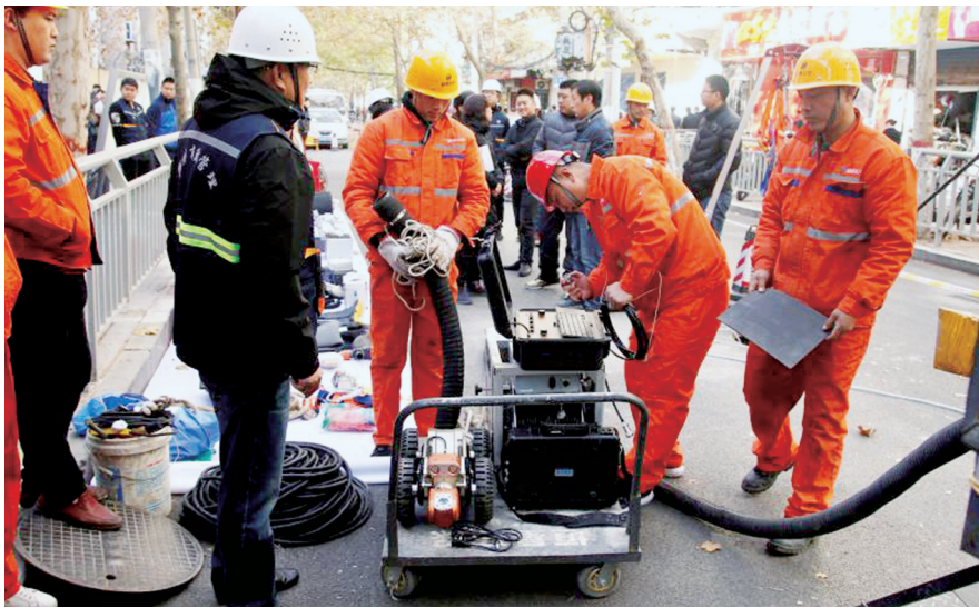
东里路污水管道非开挖修复施工
