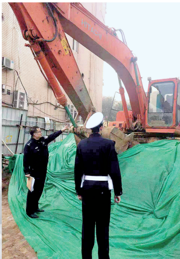
“工地警长”查扬尘
