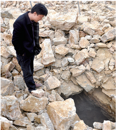
挖开后的溶洞口
